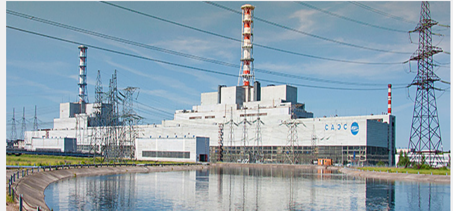
Smolensk Nuclear Power Plant
