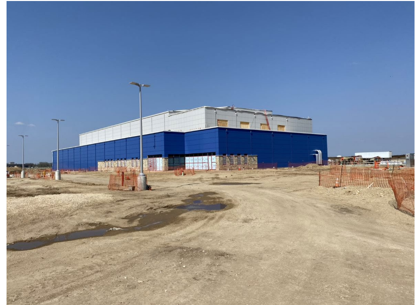
SHINE Construction Site in May 2022
