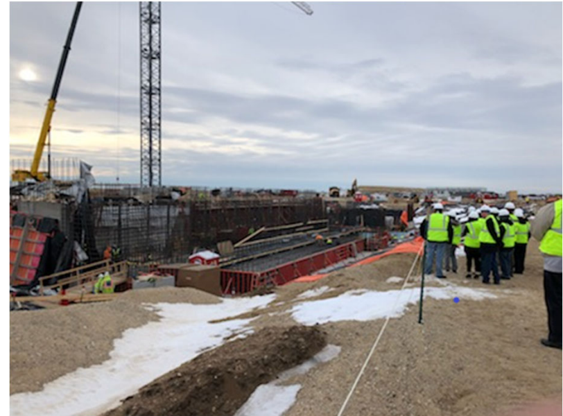
SHINE Construction Site in February 2020
