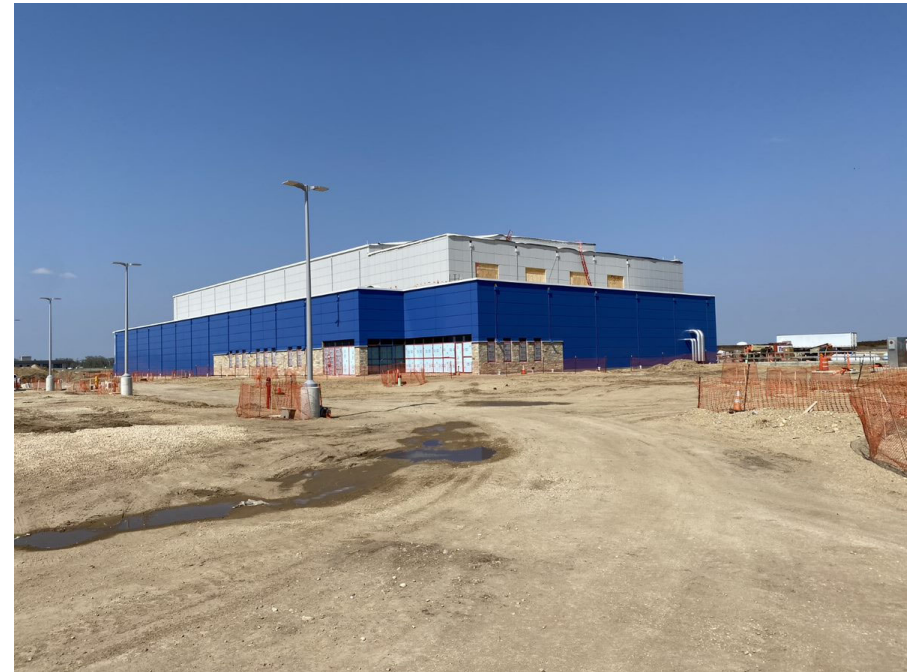
SHINE Construction Site in May 2022
