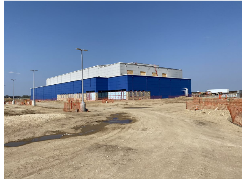
SHINE Construction Site in May 2022
